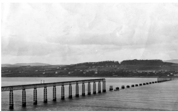
3 Long shot of the collapsed high girders section of the bridge, with twelve pier platforms almost completely swept off their high towers
