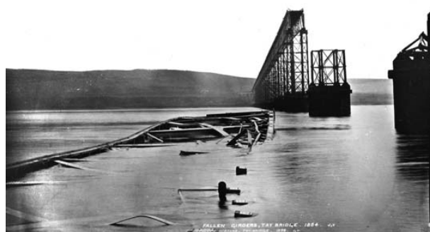
5 Side of the high girders seen at low tide. The girders were found almost intact close to the pier bases, and laid out in a wave form alongside the high section of the bridge
