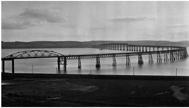
1 The Tay Bridge just after completion, showing the centre or 'high girders' section needed to allow passage of high masted sailing ships upstream along the river to Perth (clearance was about twenty-seven metres at high tide). Some finishing work was still being performed on the bridge, judging by the staging and ladders seen at various points
